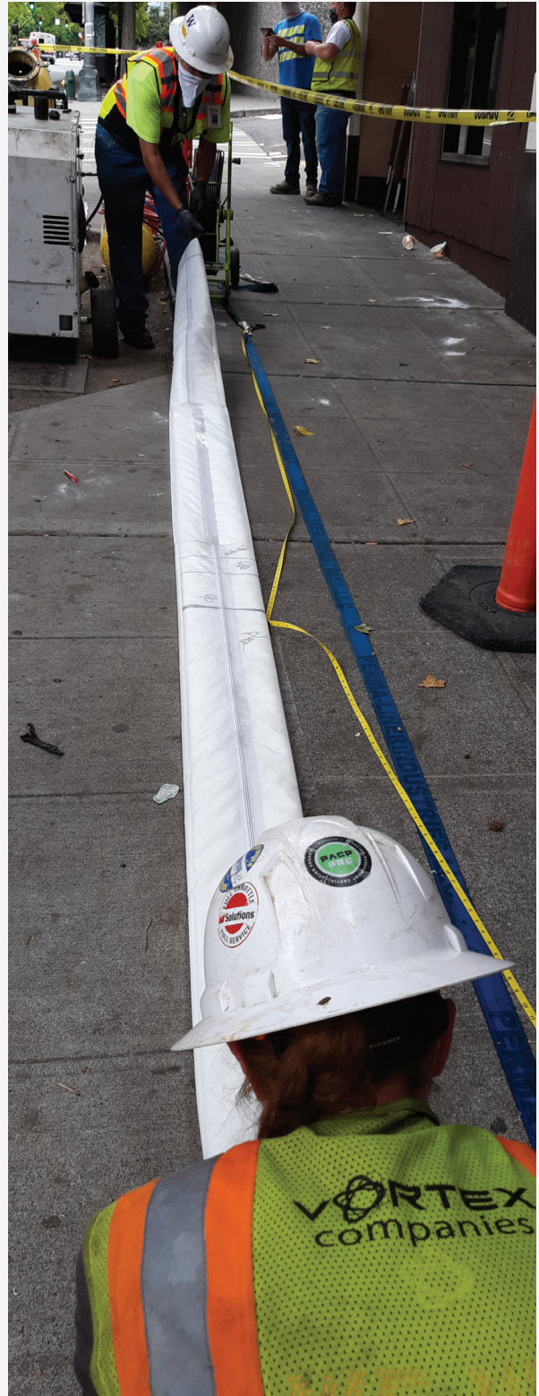
CIPP liner preparation prior to insertion into the lateral.
