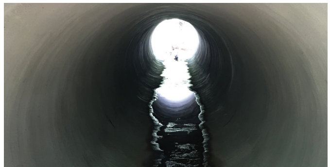
QLS GeoKrete was spray-applied, then troweled to achieve a smooth consistent thickness.
