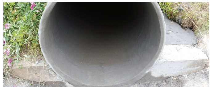
QLS GeoKrete was spin-cast for a smooth, structural and corrosion resistant finish.
