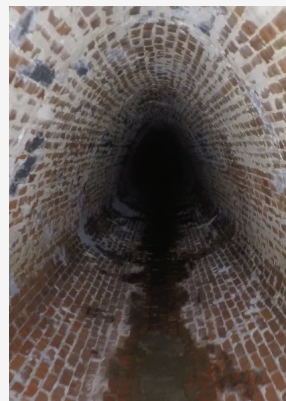
Before: Egg shaped brick outfall.
