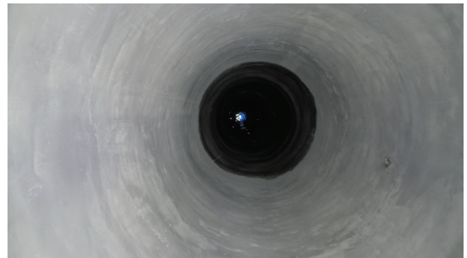
Manhole after QLS GeoKrete lined.
