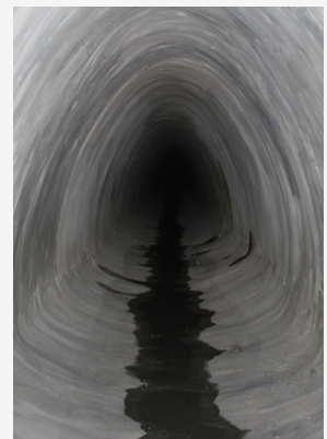
After: Outfall lined with QLS GeoKrete.
