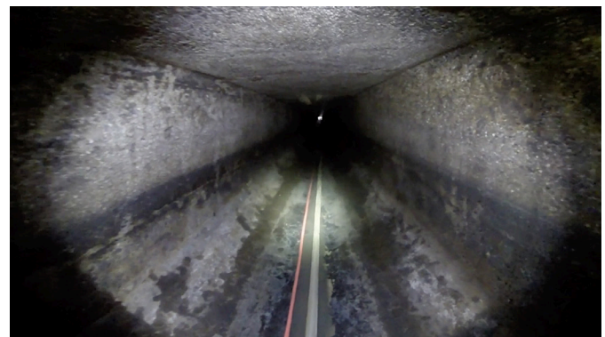
Box Culvert prepped for lining.
